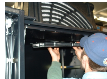
INSTALL AIR DEFLECTOR OVER OUTLET
