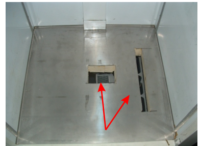
CUT INLET AND OUTLET AIR HOLES
